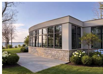
LAKE MICHIGAN SHORELINE Steel Windows Highland Park, IL
